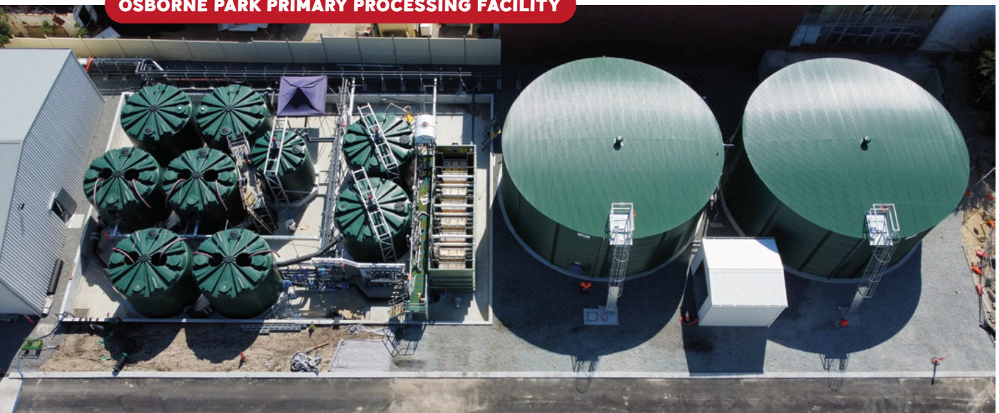
Water recycling and treatment plant, Primary processing facility, Western Australia
